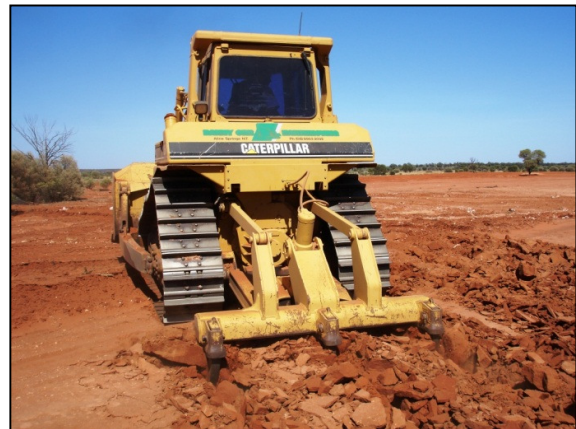
Example 3: Ripping scalded area across the slope
