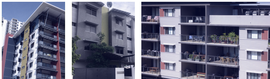
Fig 6 (left): example of a stepped wall. Fig 7 (middle) example of an expressed stairwell. Fig 8 (right): example of recessed balconies
