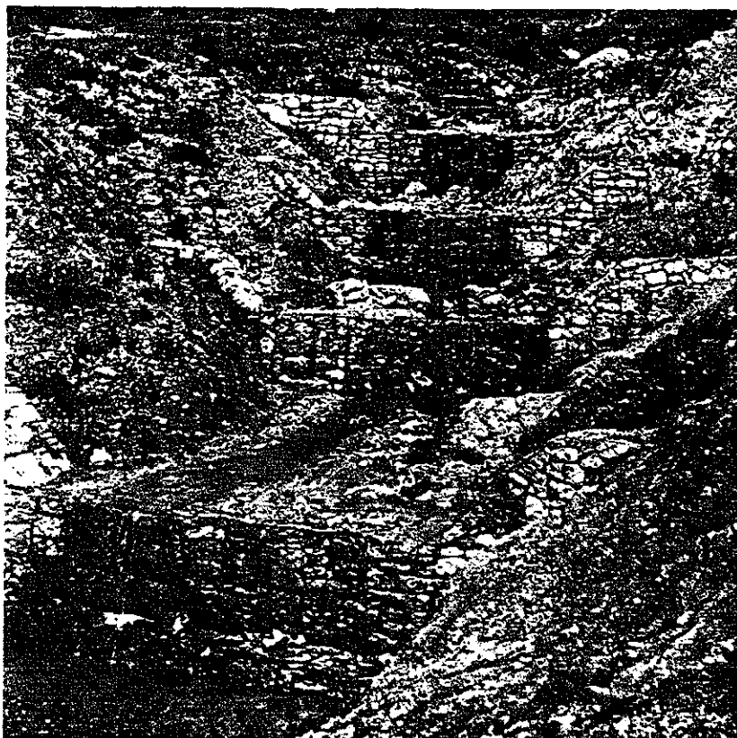
A series of small check dams preventing erosion in a gully.
