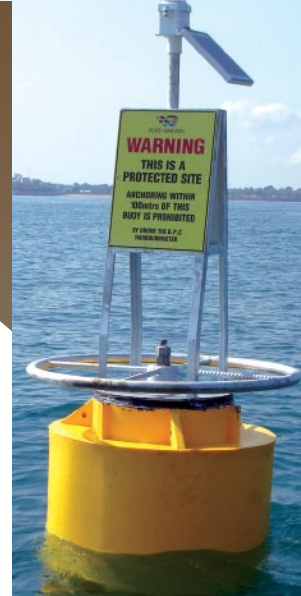
Mooring buoy on A65-115
