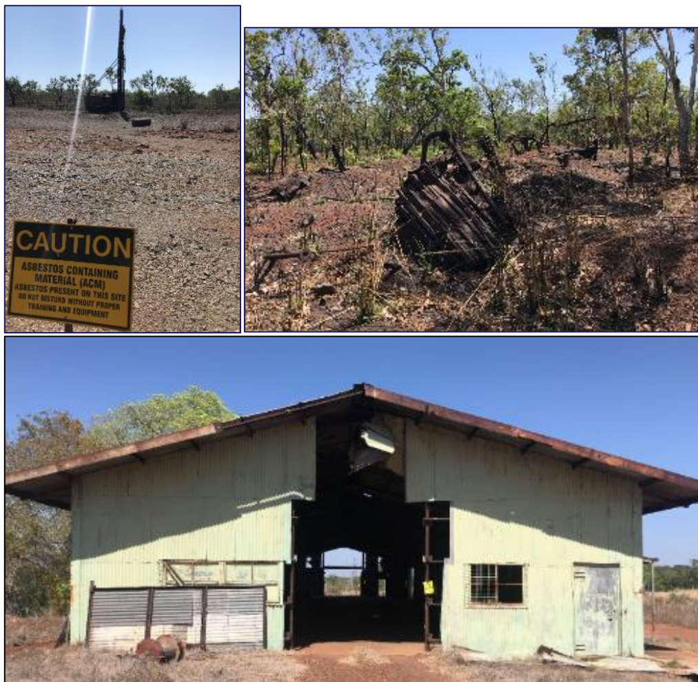
Figure 6-15: Examples of Asbestos Containing Materials (ACMs) on the former Rum Jungle Mine site
