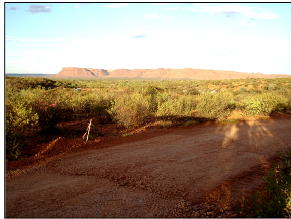
Picture 2: Whoa-boys at strategically placed intervals remove any concentrated runoff from the road.
