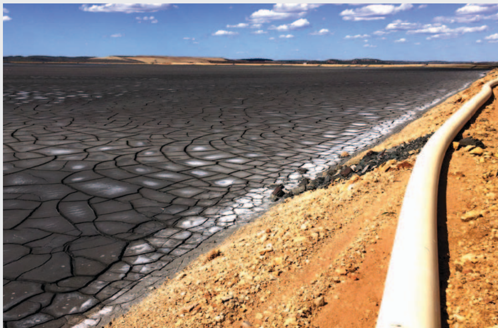
TSF Cell 2 showing most materials being moist with only minor drying at edges
