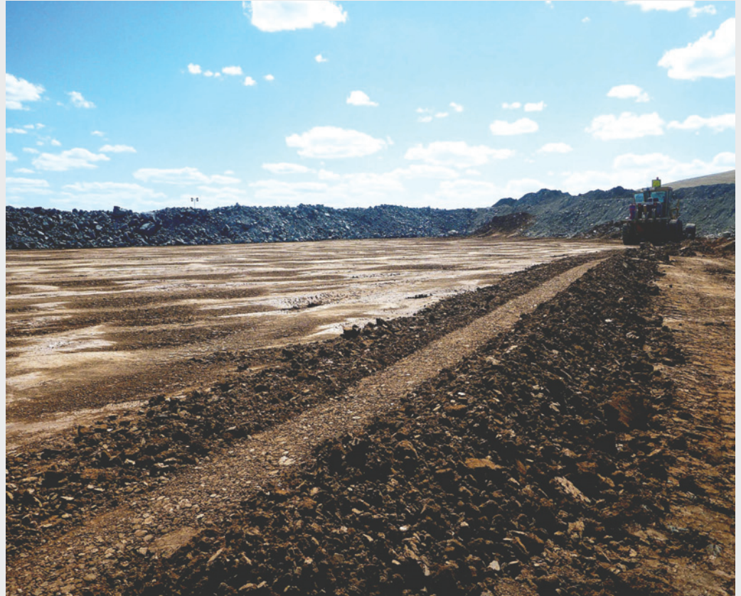
NOEF compacted base with waste rock placed over top
