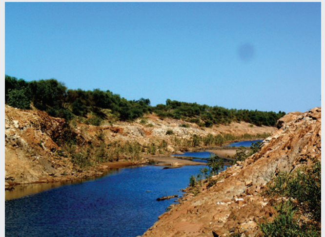
Mid-section of the diversion channel, where there is most erosion
