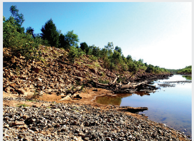
Downstream part of the diversion channel, showing large woody debris installed to create habitat and reduce erosion
