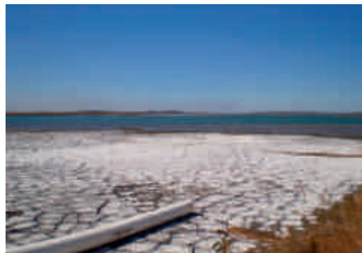
Tailings 'beach' recently deposited at the edge of TSF Cell 2, with excess water in the background - Photo taken in May, 2011.
