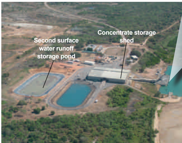
Aerial photograph of the Bing Bong Port Facility. Ore concentrate is stored in the large shed on site until it is loaded onto the Aburri Barge (photo right). As show above, a second surface runoff pond was constructed at Bing Bong in 2010 to store the large volume of runoff water from the site during the wet season. This runoff water is potentially contaminated with concentrate dust which escapes from the storage shed.
