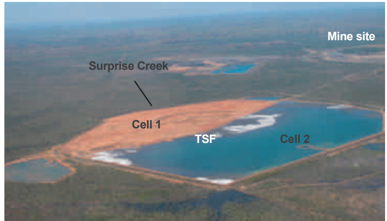
Aerial view of the Tailings Storage Facility (TSF) Cells 1 and 2. Cell 1 has now been covered with a clay to suppress tailings dust. Cell 2 is receiving tailings waste from the Mine, but was also storing more water than it should in May 2011
