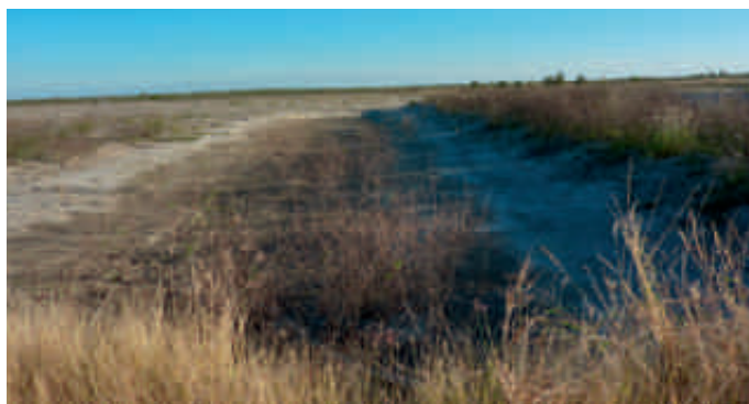
Above: Series of photographs taken in 2009, 2010 and 2011, showing the outer toe of the spoil ponds, with the spoon drain subsequently installed in late 2009 to redirect saline seepage out to sea.
