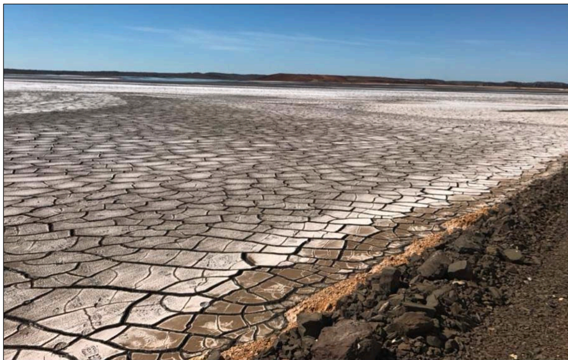
Plate 4.8 – Salt Crusting on TSF Surface
