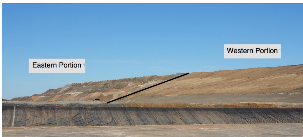
Plate 4.4 – Northern Face of the NOEF Showing Flattened Western Portion Ready for Advection Barrier and Eastern Portion Still to be Flattened
