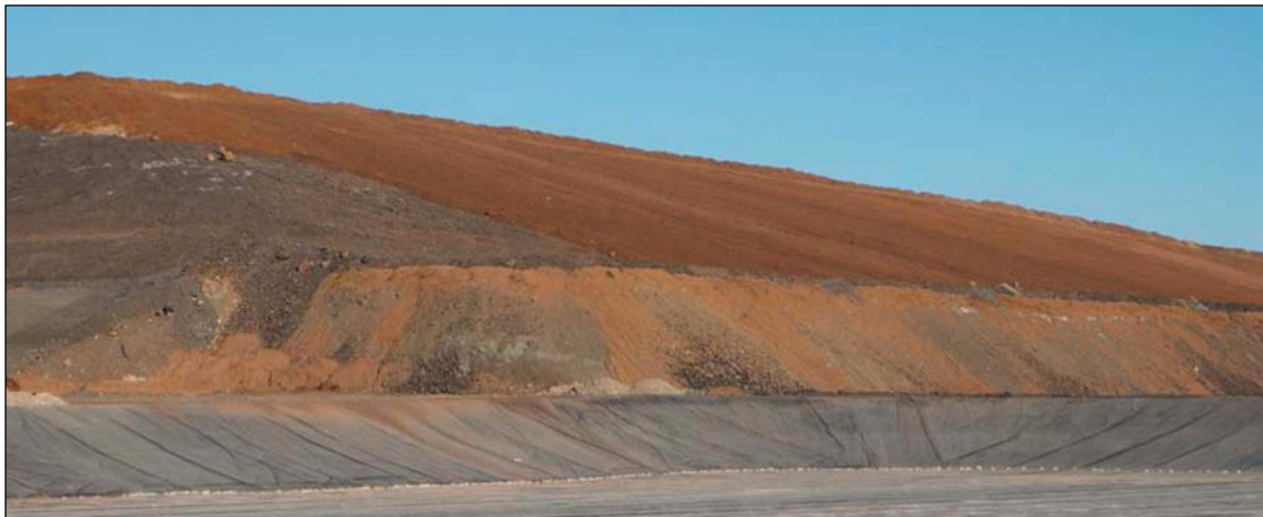
Plate 4.5 – Advection Control Layer on Western Face of NOEF
