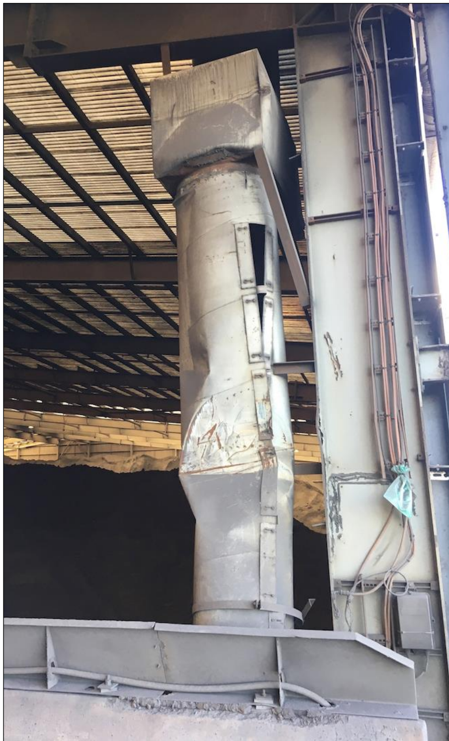
Plate 4.14 – Dust Vent at Bing Bong Loading Facility Concentrate Shed
