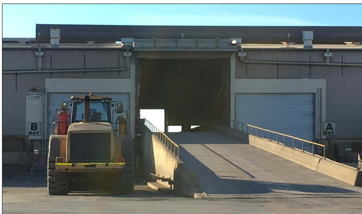
Plate 4.13 – Replaced Side Doors at Bing Bong Loading Facility Concentrate Shed
