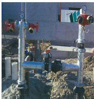
“H” Fire + Sprinkler Booster
