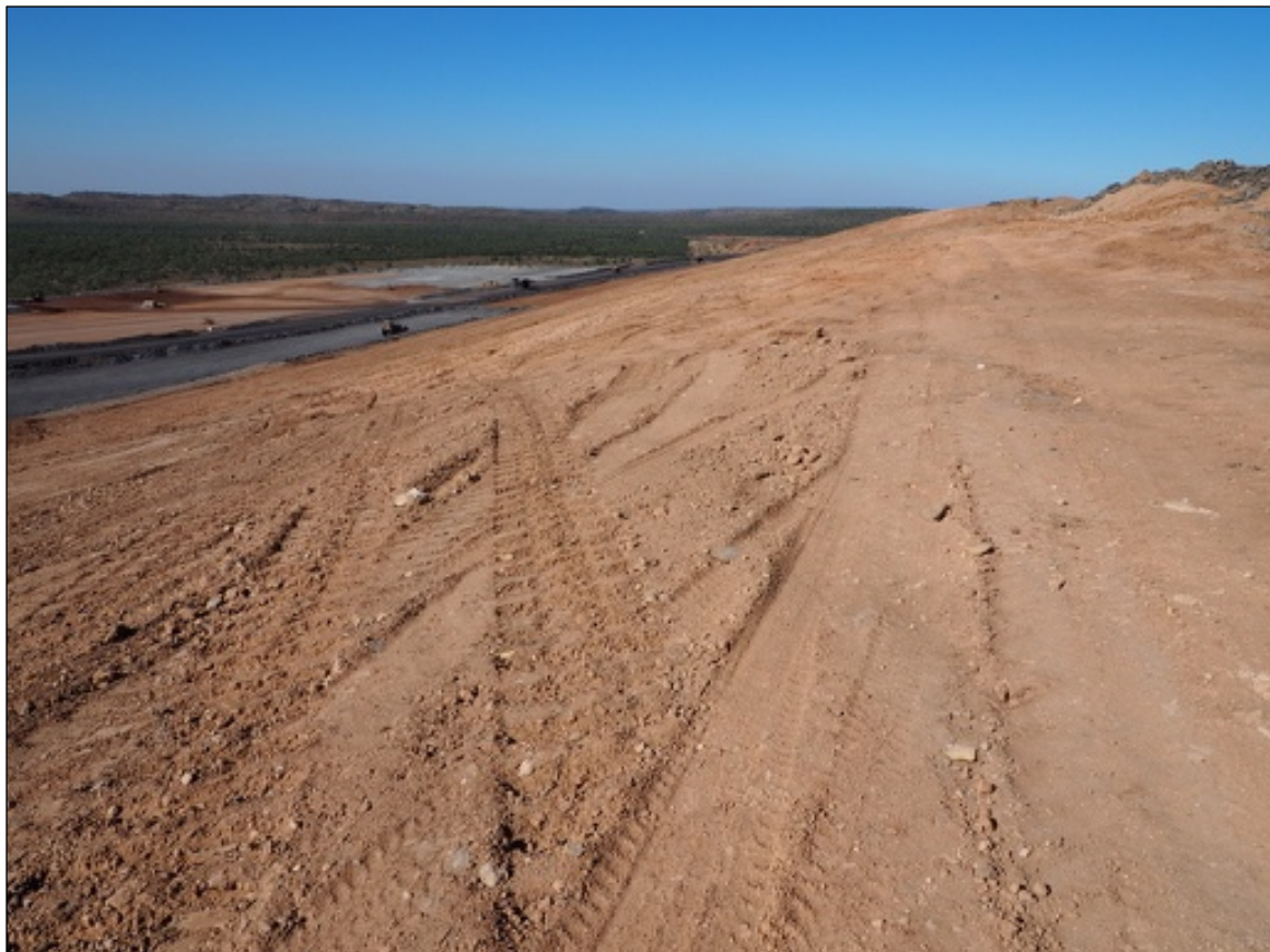
Plate 4.3 – Interim 0.5 m Advection Barrier Between the Older NOEF Dump Area and CW Stage
