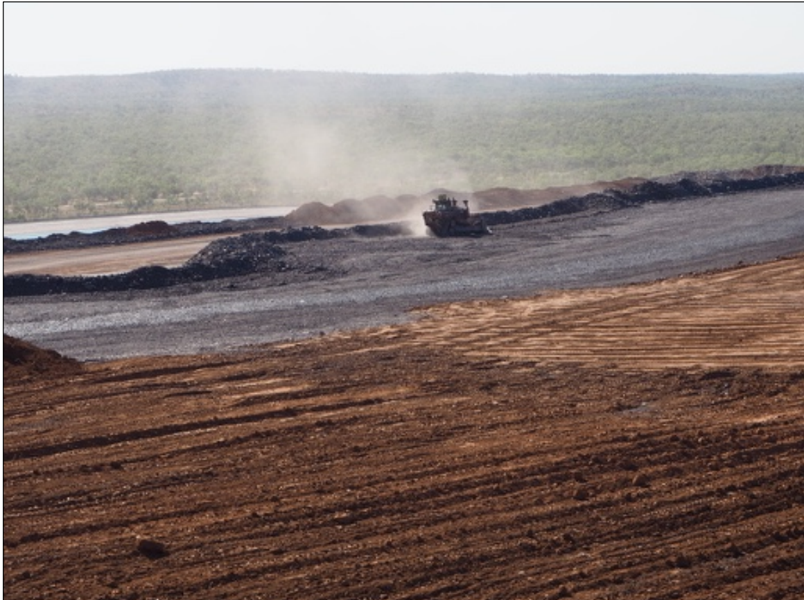
Plate 4.1 – Example of Dozing PAF Cell Placement in CW Stage of the NOEF
