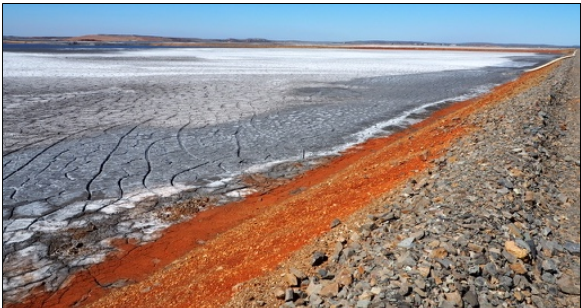
Plate 4.6 – TSF Cell 2 Showing Salt Crusting on Surface
