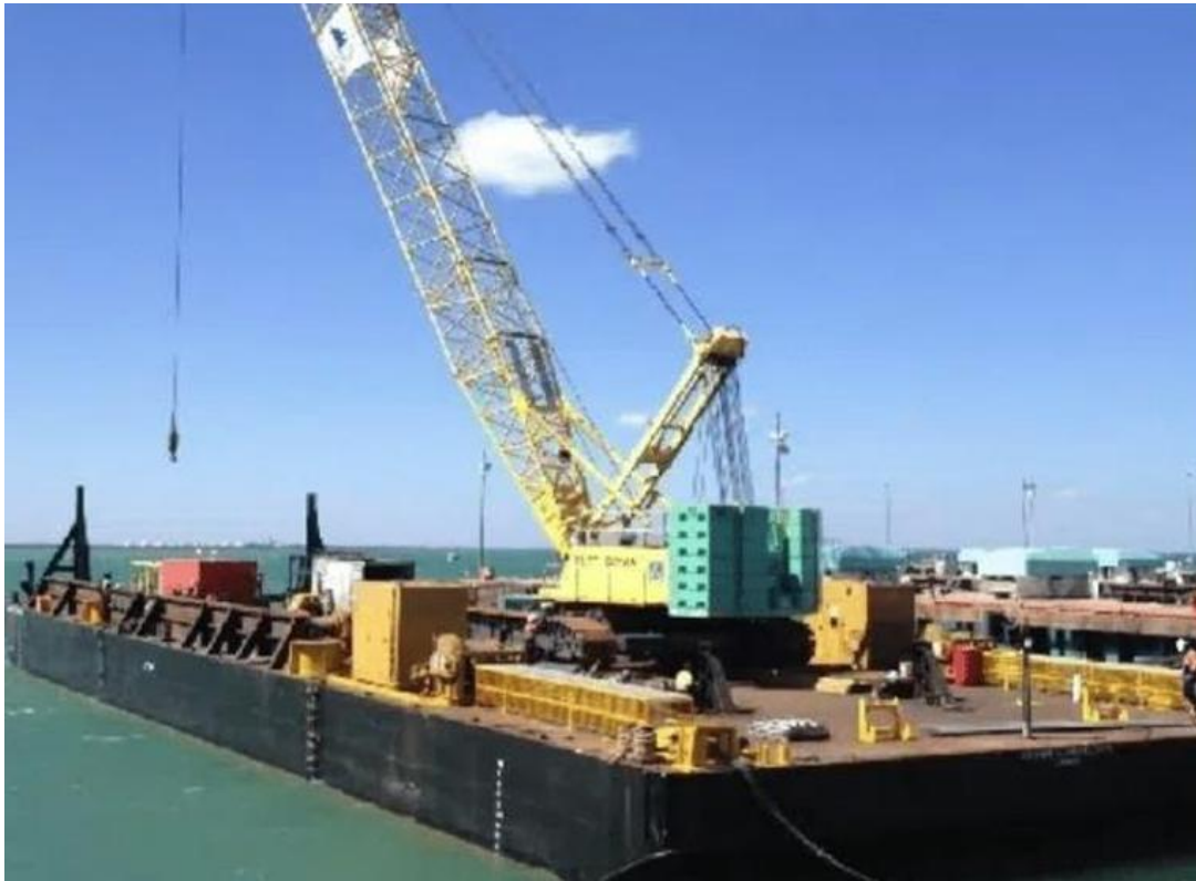
Figure 4: Construction Barge - Arnhem Constructor
