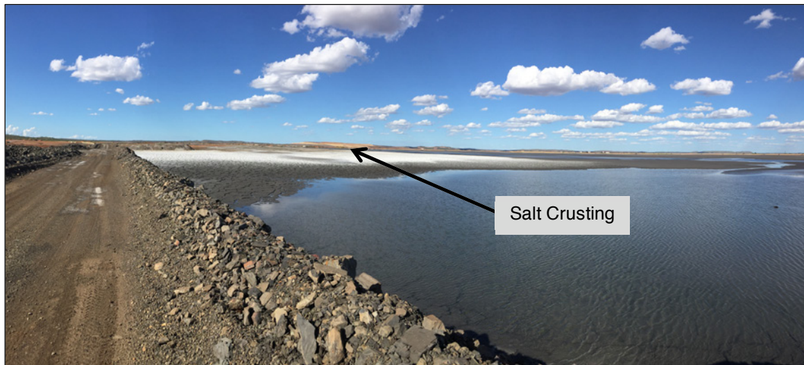
Plate 4.7 –TSF Cell 2 Showing Salt Accumulation on Tailings Surfaces East of the Decant Causeway
