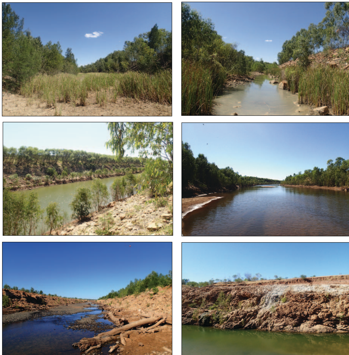
Clockwise from top left: 1. Barney Creek diversion channel at the confluence with Surprise Creek (SW18) looking up Barney Creek. 2. At the same location looking downstream. 3. Good revegetation at the upstream end of the McArthur River diversion channel. 4. Sparse vegetation along the rocky walls of the middle section of the McArthur River diversion channel. 5. Large woody debris, sediment deposits and low vegetation at the downstream end of the McArthur River diversion channel. 6. Reasonable low water shoreline revegetation towards the upstream end of the McArthur River diversion channel.
