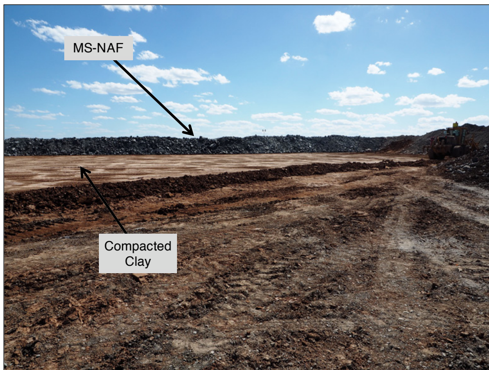
Plate 4.3 – Compacted Clay Layer (600 mm) Constructed on LS-NAF Materials on the South Side of the NOEF, with MS-NAF Materials Being Paddock Dumped over the Top
