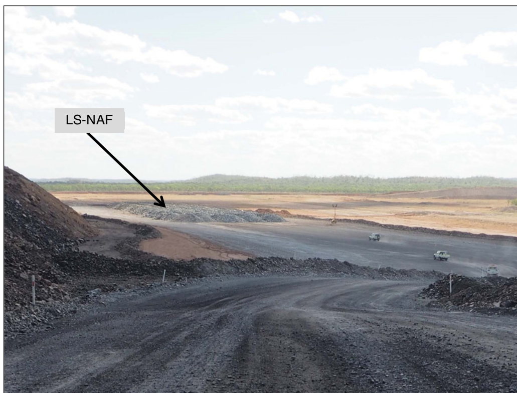
Plate 4.3 – Compacted Clay Layer (600 mm) Constructed on LS-NAF Materials on the South Side of the NOEF, with MS-NAF Materials Being Paddock Dumped over the Top
