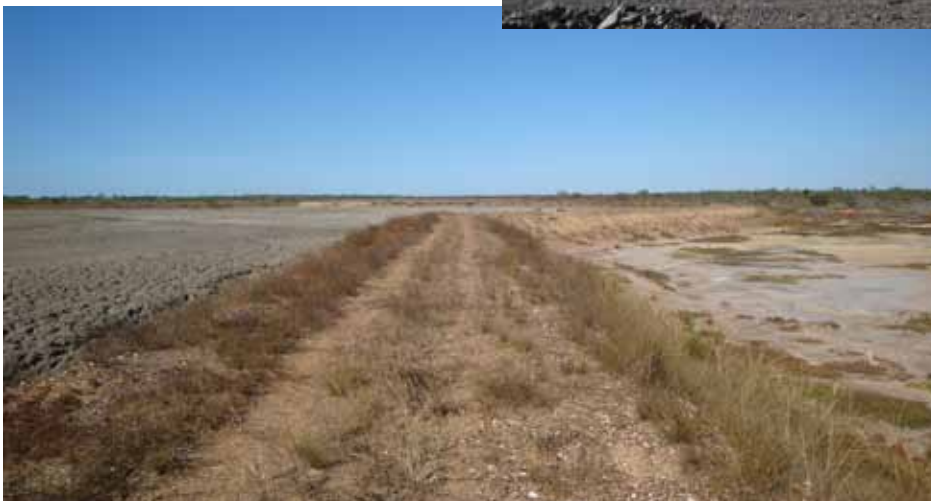
Dredge soil pond wall separating the dredge material (left) from the surrounding land.
