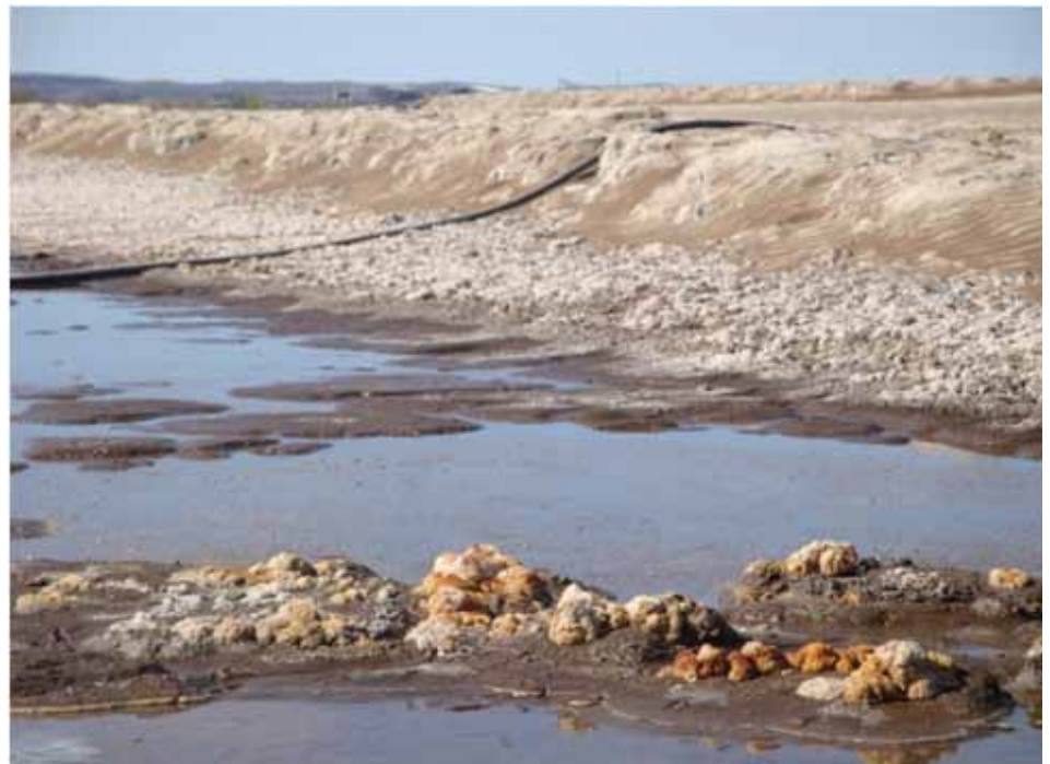
Tailings seepage draining from the foot of Tailings Storage Facility Cell 1 into Surprise Creek (above), and Iron sulfate salts at the surface of Cell 1 (below) (Photo June 2009, Independent Monitor).
