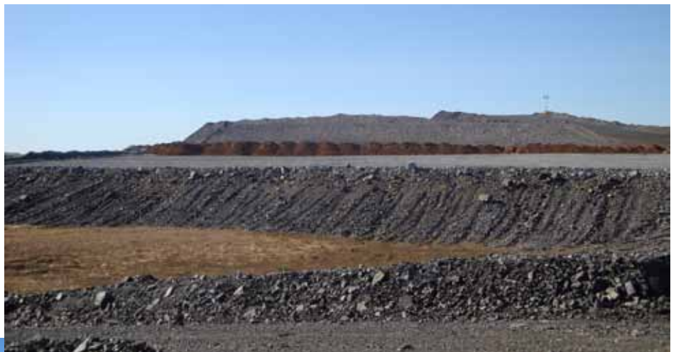
The Overburden Emplacement Facility where waste rock from mining is placed (Photo June 2009, Independent Monitor).
