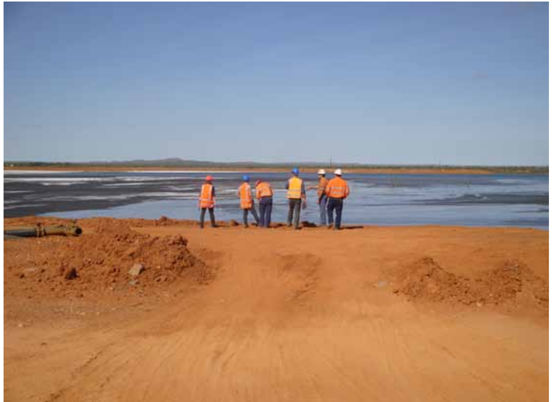
The Independent Monitor and MRM inspecting the clay layer covering the Tailings Storage Facility (foreground) with fresh tailings in the distance. (Photo by Independent monitor, June 2009)
