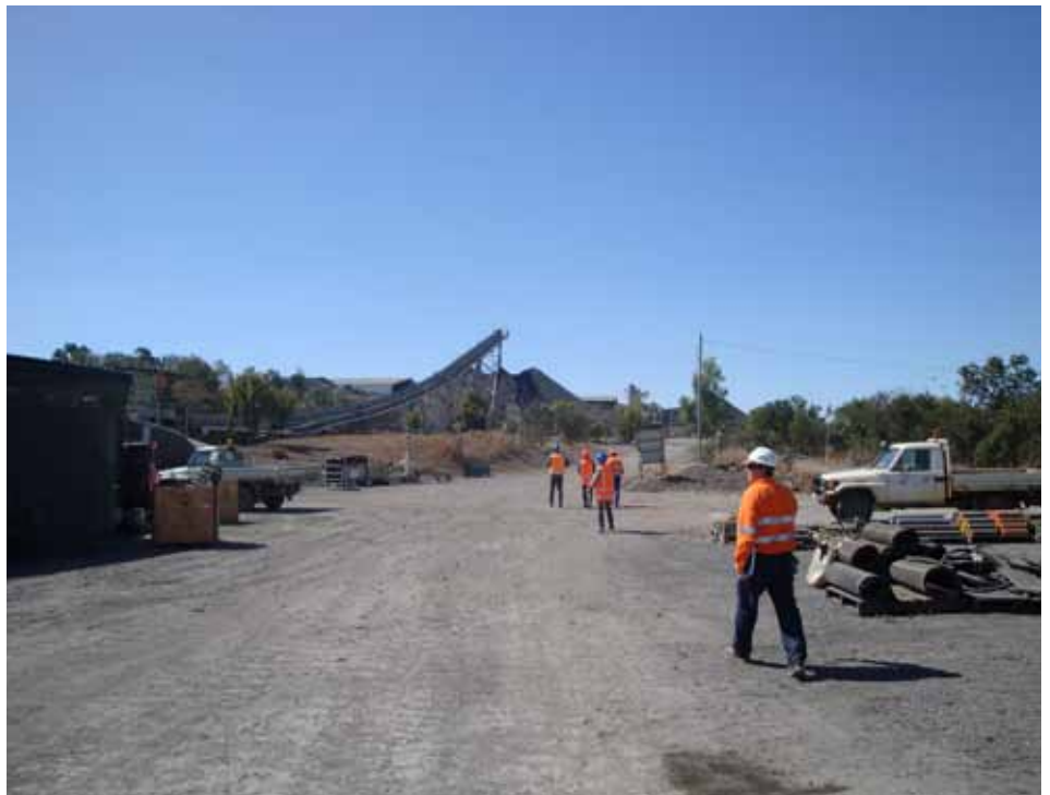
Run of Mine Pad at the mine site (Photo June 2009, Independent Monitor).
