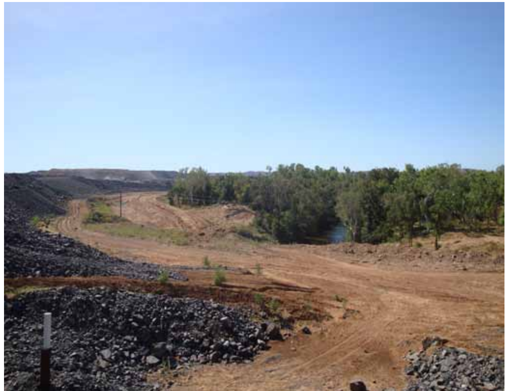
(Above) Cut-off section of the old McArthur River at the mine site (Photo June 2009, Independent Monitor).
