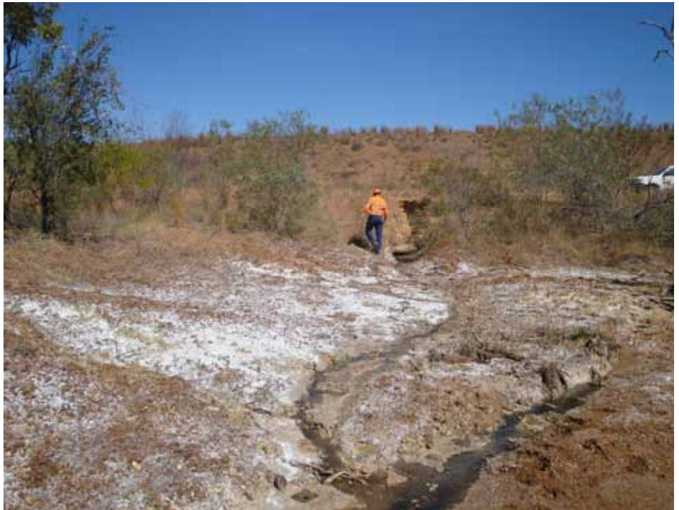
Tailings seepage draining from the foot of Tailings Storage Facility Cell 1 into Surprise Creek (above), and Iron sulfate salts at the surface of Cell 1 (below) (Photo June 2009, Independent Monitor).
