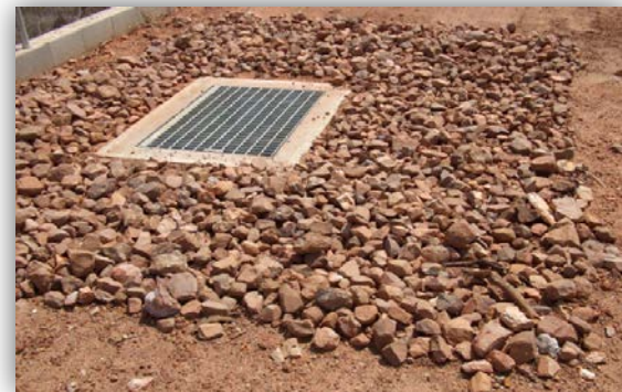
Example of inlet pit protection. Grated pits can also be wrapped in geofabric or sediment fence material.
