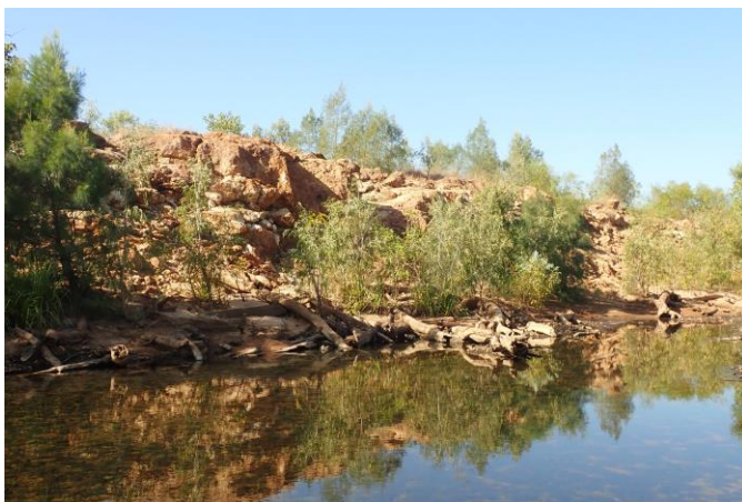
Photo 10: Example of medium woody debris placed to improve macroinvertebrate assemblages along the McArthur River Diversion Channel.
