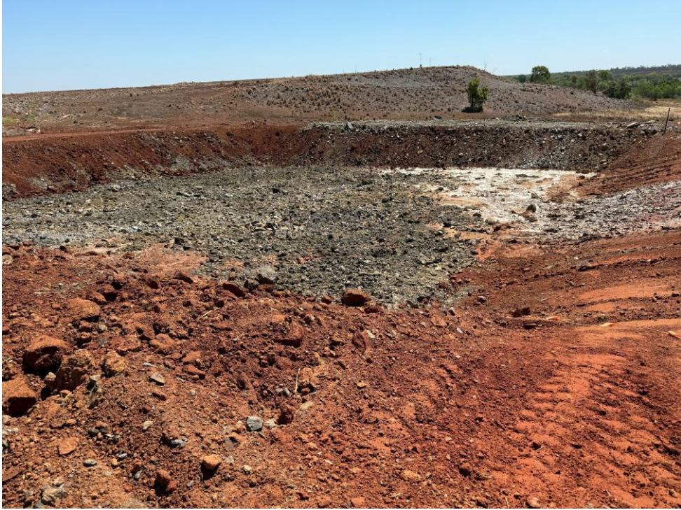
Plate 7 Co-disposal pit on Main Waste Rock Dump
