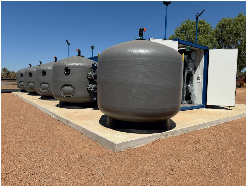
Plate 9 Part of the Surface Water Treatment Plant
