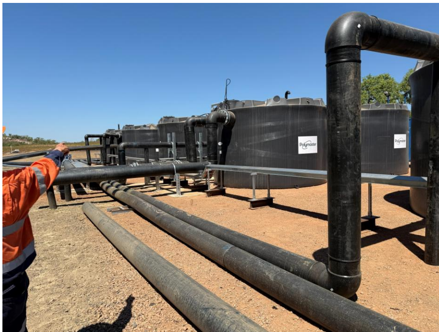
Plate 8 Part of the Surface Water Treatment Plant
