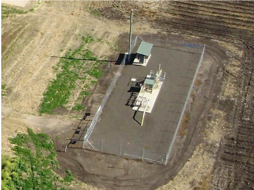
Figure 3.5 General photo showing an above ground facility
