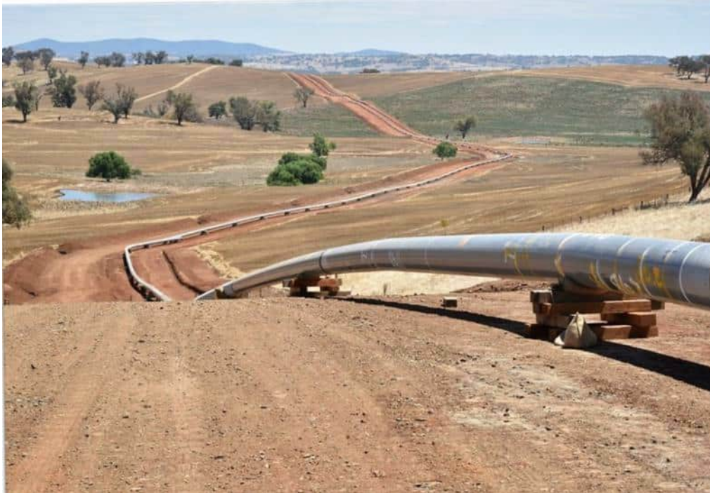
Figure 3.15 ROW during construction
