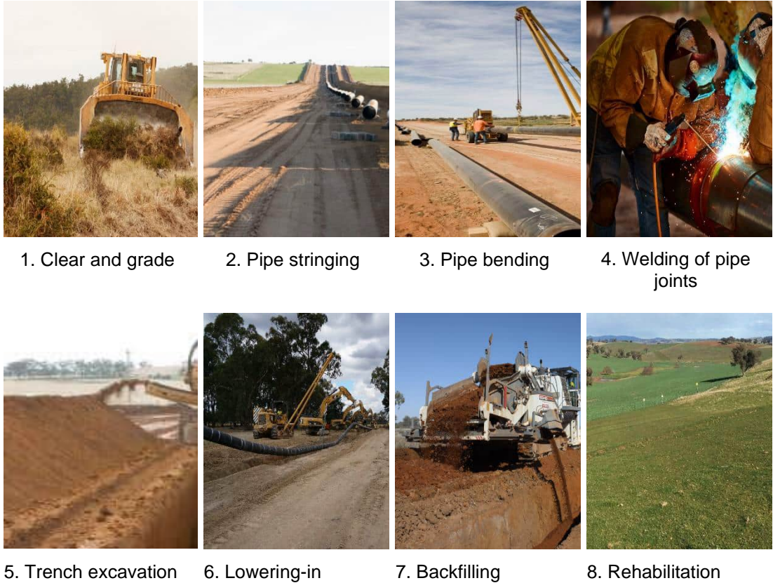
Figure 3.11 Pipeline construction sequence
