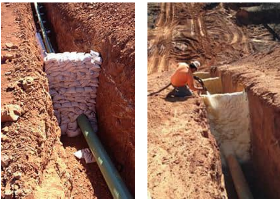
Figure 3.14 Example of trench breakers
