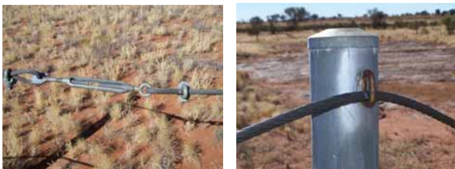
Figure 5. Close-up of cable fastening and fixture for the 'cable fence'
