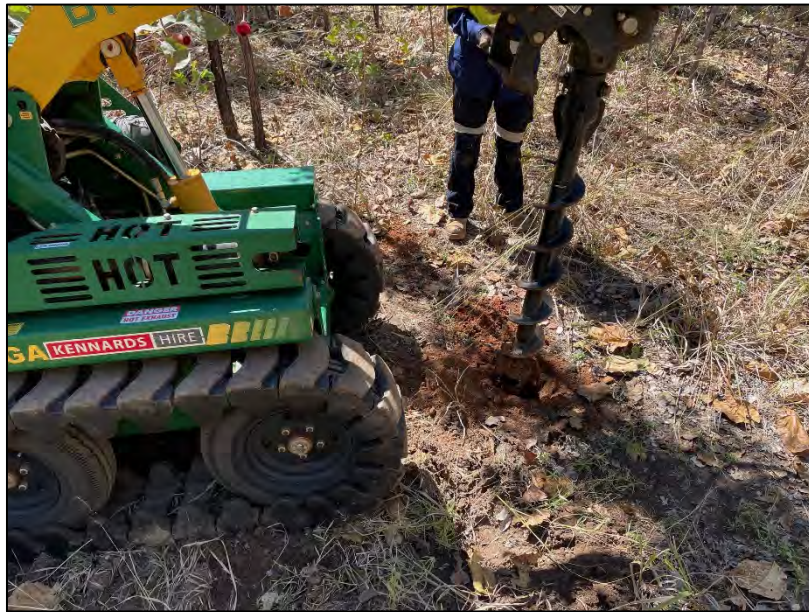
Figure 2-2. Photograph of Tracked Mini Loader with auger
