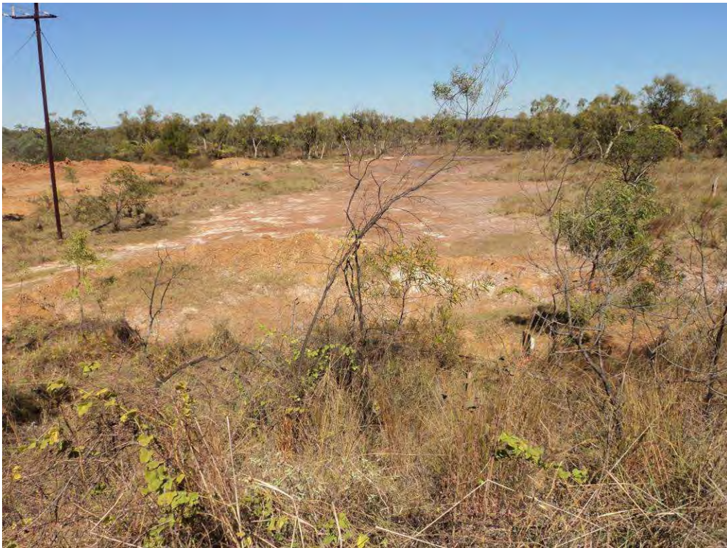
Plate 30 Seepage causing salt precipitation in an area south of the TSF Cell2, downstream from the 'contaminated waste area' of the WMD.
