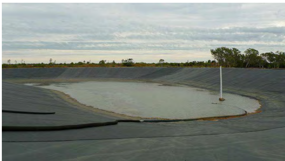
Plate 2 A third surface water runoff pond has been installed since 2011. This additional storage pond increases MRM's capacity to store potentially contaminated surface runoff water at the Bing Bong Port facility through the Wet Season.
