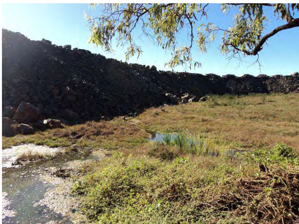
Plate 39 Area of seepage observed from the north eastern toe of the OEF. This seepage is collected in a downstream pump.
