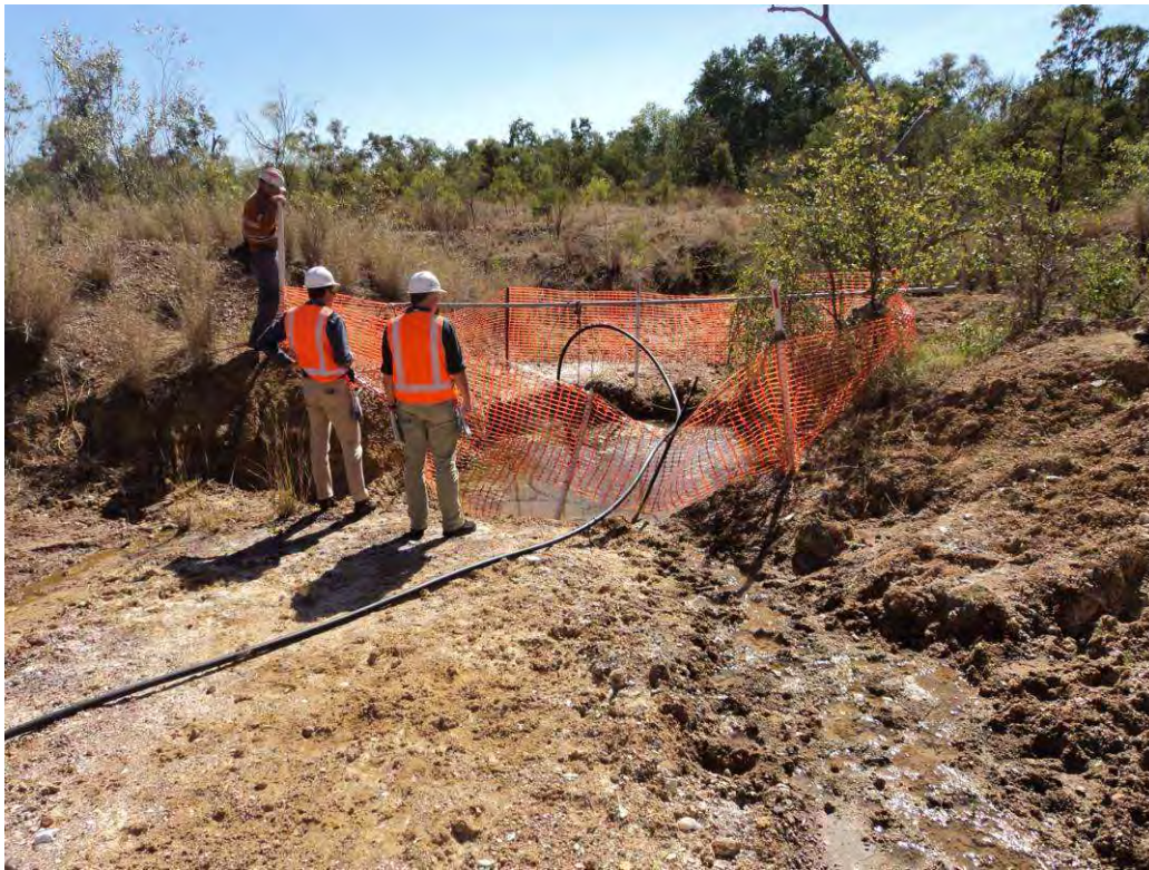
Plate 29 Seepage flowing from the toe of TSF Cell1 embankment towards Surprise Creek is captured within a sump, shown above.
