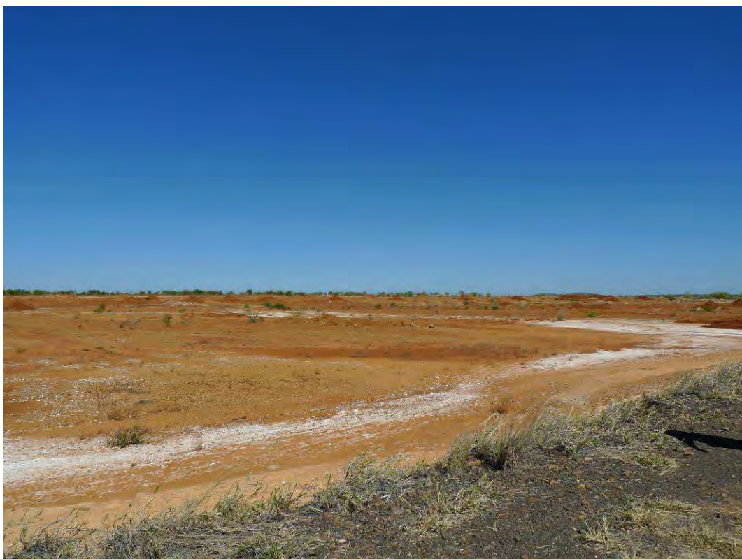
Plate 31 Salt Precipitation on clay capping of Cell 1, May 2012.
