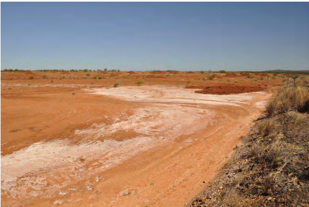
Plate 20 Sparse natural revegetation of areas of TSF cell 1 with no topsoil observed during 2012 site inspection. This area allows run-off to flow around the edge of the TSF to a collection point for pumping to TSF cell 2. Clay top soil piles will be dispersed to control area of erosion on the surface of TSF cell 1.
