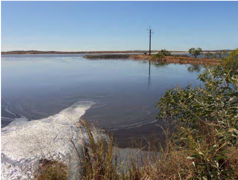
Plate 33 Tailings deposition along southern embankment of Cell 2.
