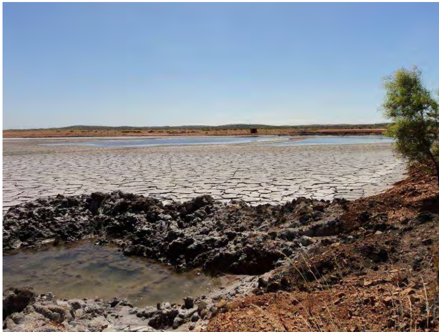
Plate 34 Recently (6 months) deposited tailings along eastern wall, which had recently been disturbed because of geotechnical testing (CPT).
