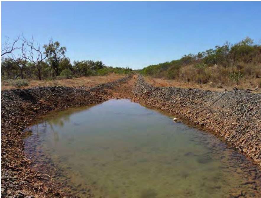
Plate 36 Sump and drain along eastern embankment of Cell 2 near Little Barney Creek.
