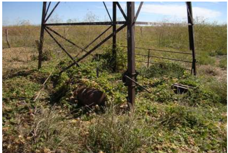
Plate 4. Lower section of the tower with bore hole directly in the centre.
