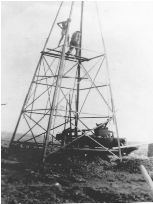
Plate 1. Erecting the Comet Windmill at No.1 Bore, Ucharonidge Station (Source: Coral Beebe).
