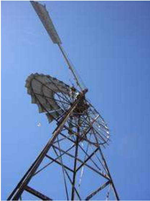
Plate 3. Upper section of the tower showing the windmill head and fan. Note the tail has been positioned to stop the fan moving into the wind.
