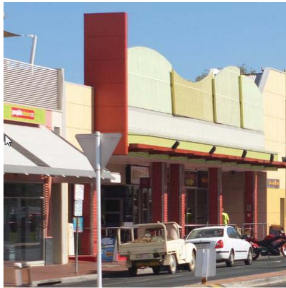
Figure 13 – Example of effective screening of multi-level car parking with active street frontage
