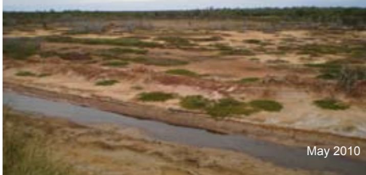
Top: Salt-affected land and vegetation outside of the Bing Bong Dredge Spoil ponds in June 2009. Bottom: The same area in May 2010 after the installation of a perimeter spoon drain, which is seen in the foreground. Vegetation is seen to be regenerating outside of the spoon drain.
