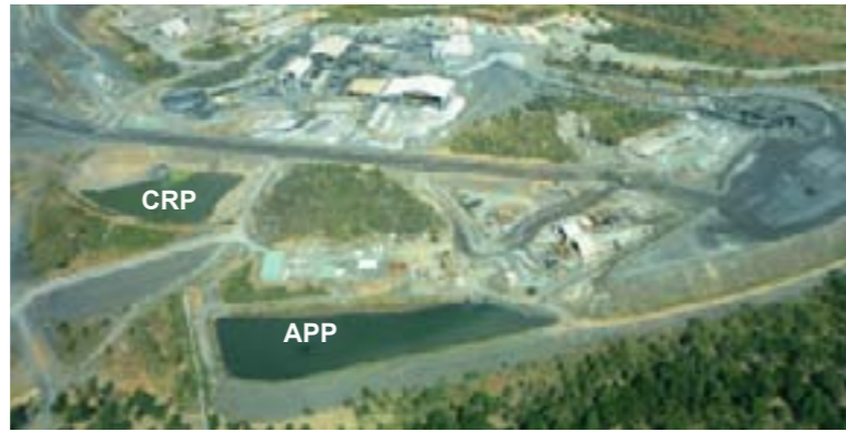
Monitoring of artificial surface waters is undertaken at all water dams across the Mine site and at Bing Bong on a monthly basis. The above photograph shows the Concentrator Runoff Pond (CRP) and Anti Pollution Pond (APP) at the Mine site. The 2009 data collected by MRM indicated that the CRP may be leaking, and MRM have proposed investigation and mitigation strategies in response. (May 2010).
