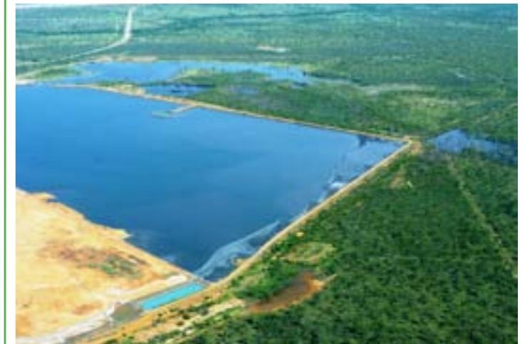
There is a large volume of water being stored in TSF Cell 2 as seen above. The water management dam (top left of the photo) receives excess water spillover from Cell 2, but the amount of water stored, in the Cell should be reduced (May 2010).
