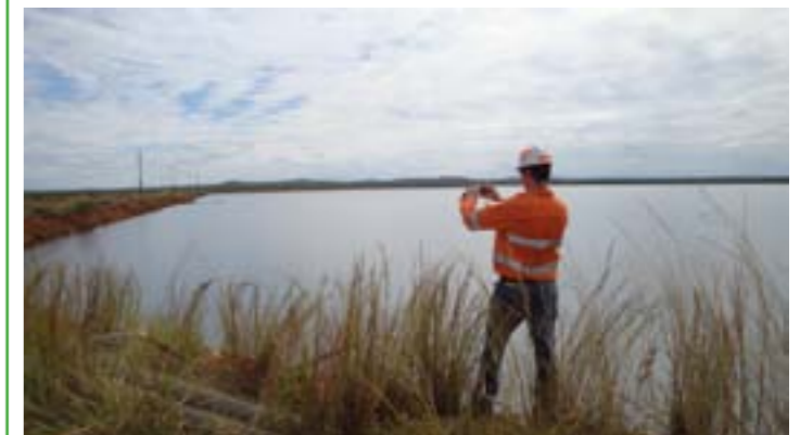
Independent Monitor team geotechnical engineer inspecting the excess water storage in TSF Cell 2 (May 2010). As seen above, at the time of our inspection, there was only approximately 1 metre of freeboard available in Cell 2. The available freeboard should be increased to reduce the risk of overtopping.
