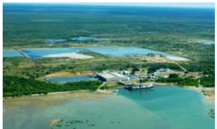
Aerial view of the Bing Bong Port Facility with the Bing Bong Port and concentrate storage shed in the foreground, and the dredge spoil ponds in the background. (May 2010).
