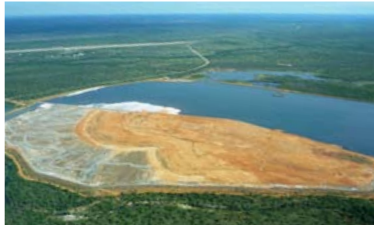
The clay capping of TSF Cell 1 was approximately 60% complete during our inspection in May 2010, as seen above. The rest of the capping is to be completed by the 2010/2011 wet season to reduce infiltration of water through the exposed tailings and reduce dust generation.
