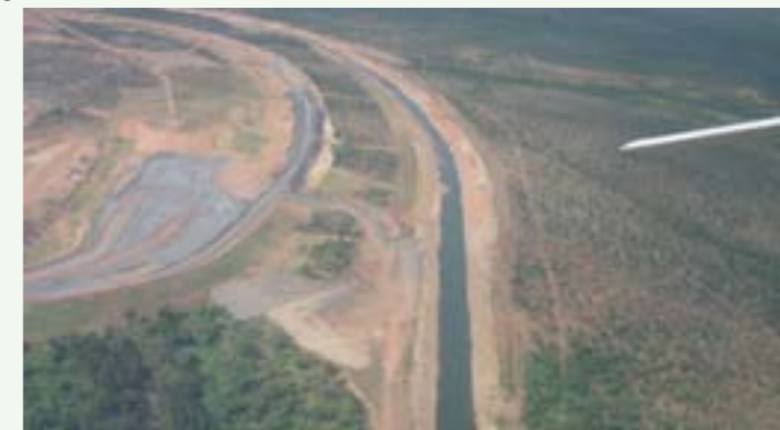
The above photograph shows the upstream end of the McArthur River Diversion, and the cut off section of the old McArthur River channel to the bottom left. During times of flood, water passes overland between the two.
