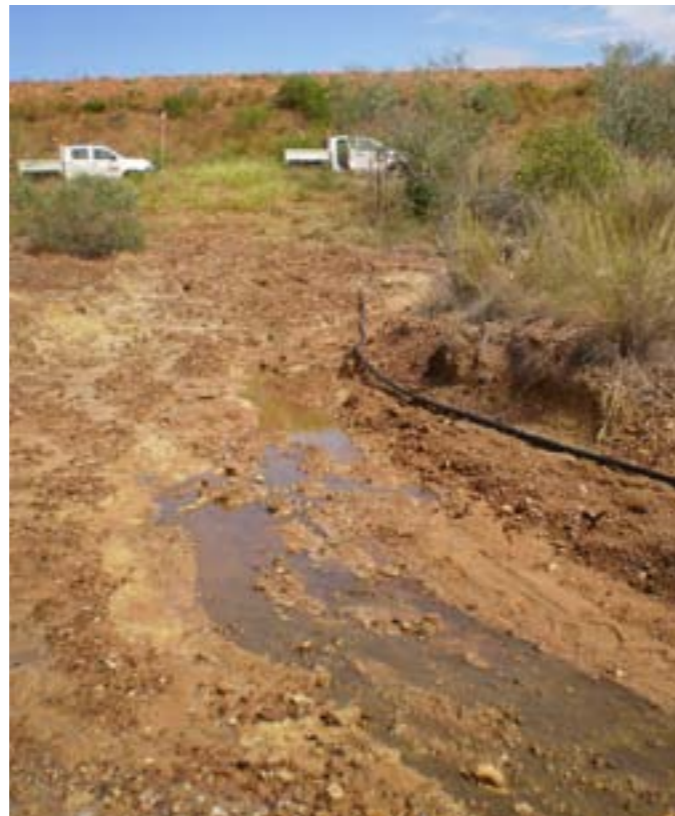
Leachate draining from the base of TSF Cell 1 towards Surprise Creek. A sump has been constructed to collect some of this leachate, but more work is needed (May 2010).
