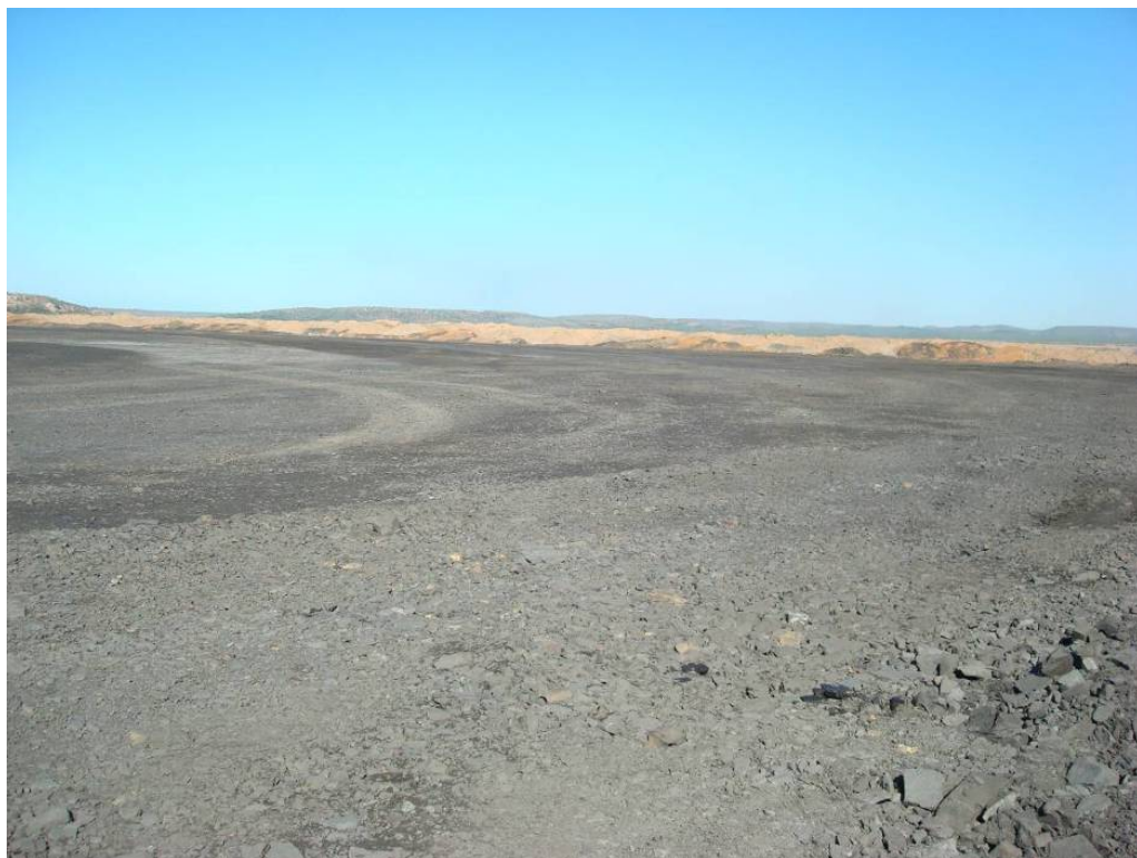
Plate 44 Top surface of OEF (PAF waste in foreground and an area clay covering in the background). Photo: Independent Monitor
