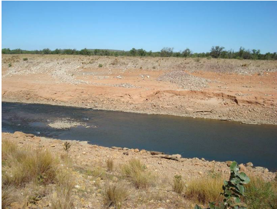
Plate 51 Minor erosion of McArthur diversion batter. Photo: Independent Monitor
