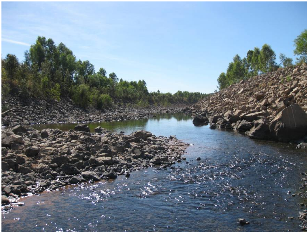
Plate 66 Looking downstream along Barney Creek diversion channel at Surprise Creek confluence. 2010 rock armouring of channel batter slope opposite Surprise Creek entry (to address 2009/2010 wet season scour) is shown in right hand portion of photo. Photo: Independent Monitor
