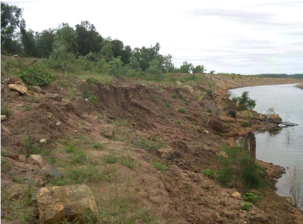
Plate 60 Example of relatively minor bank erosion in the McArthur River diversion channel taken at the same location in 2011 (top) and 2010 (bottom), showing little change). Photos: Independent Monitor.
