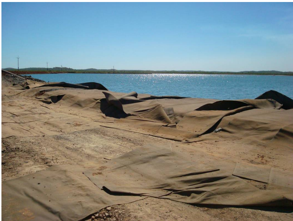
Plate 36 Temporary bund in spillway constructed of soil covered in geofabric. Photo: Independent Monitor.
