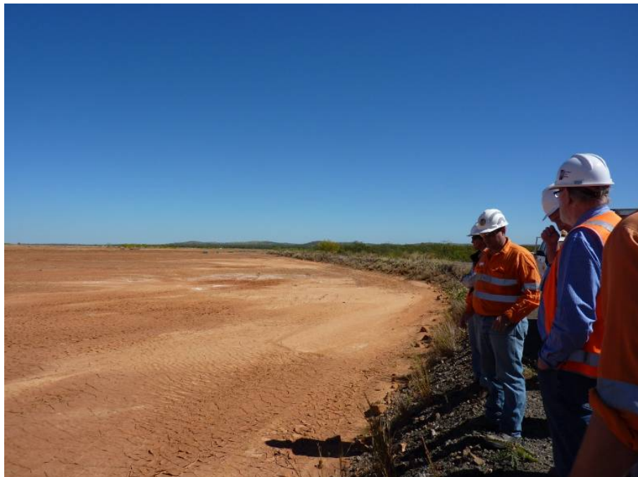
Plate 21 Clay capping of TSF Cell1. Photograph: Independent Monitor.
