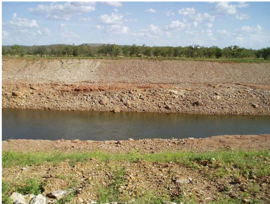
Plate 56 View of eastern batter slope scour at river channel chainage 1750m; taken March 2009. Photo: Independent Monitor
