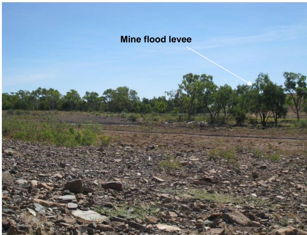
Plate 61 View of rock work placed in the foreground and background in 2010 to address scour along the overland flow path from the old McArthur River channel to the diversion channel. Photo is taken looking towards the old channel alignment. The mine levee wall can be seen behind the trees to the right. Photo: Independent Monitor
