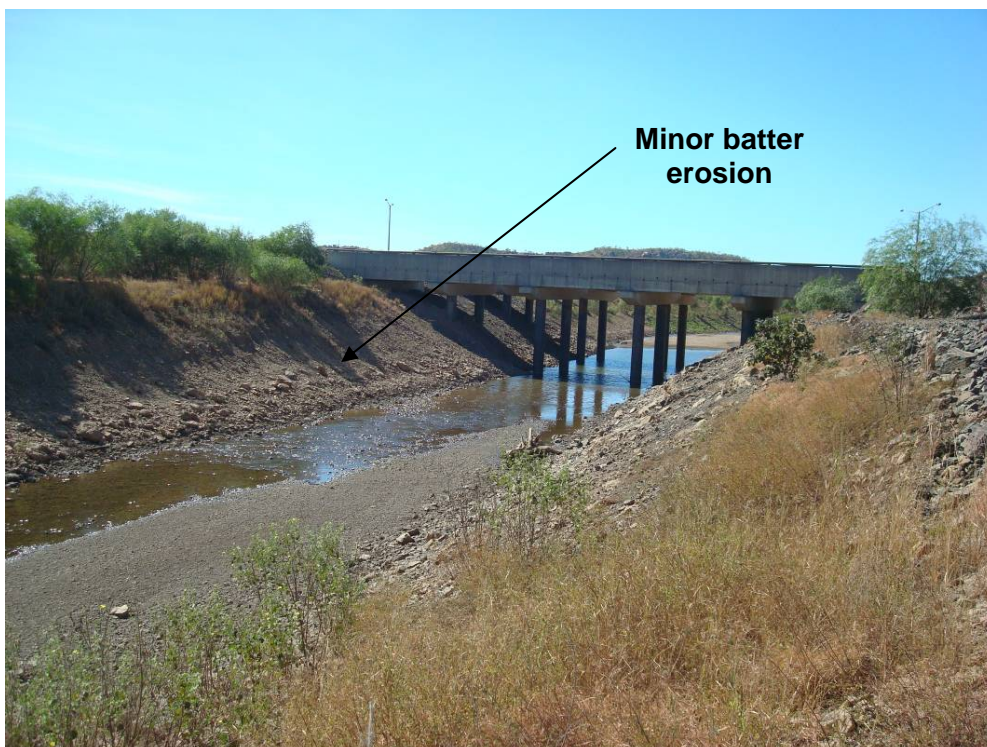
Plate 46 Barney Creek diversion channel upstream of bridge to OEF; note minor erosion of the batters. Photo: Independent Monitor
