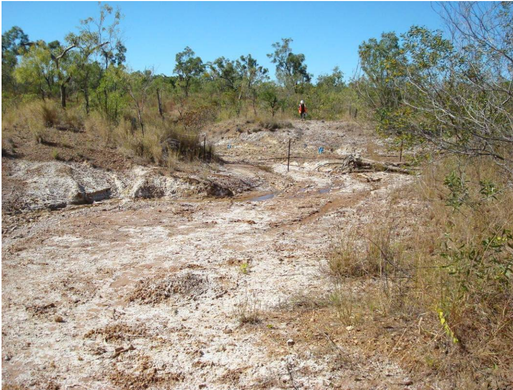
Plate 32 Extensive salt precipitation and active seepage zone downstream of TSF Cell 1 embankment toe adjacent to Surprise Creek. Photo: Independent Monitor.
