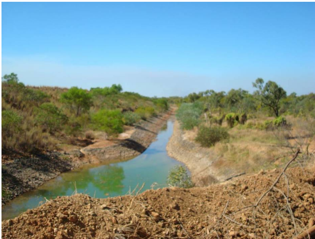
Plate 38 Eastern seepage collection drain at toe of TSF Cell 2. Photo: Independent Monitor.
