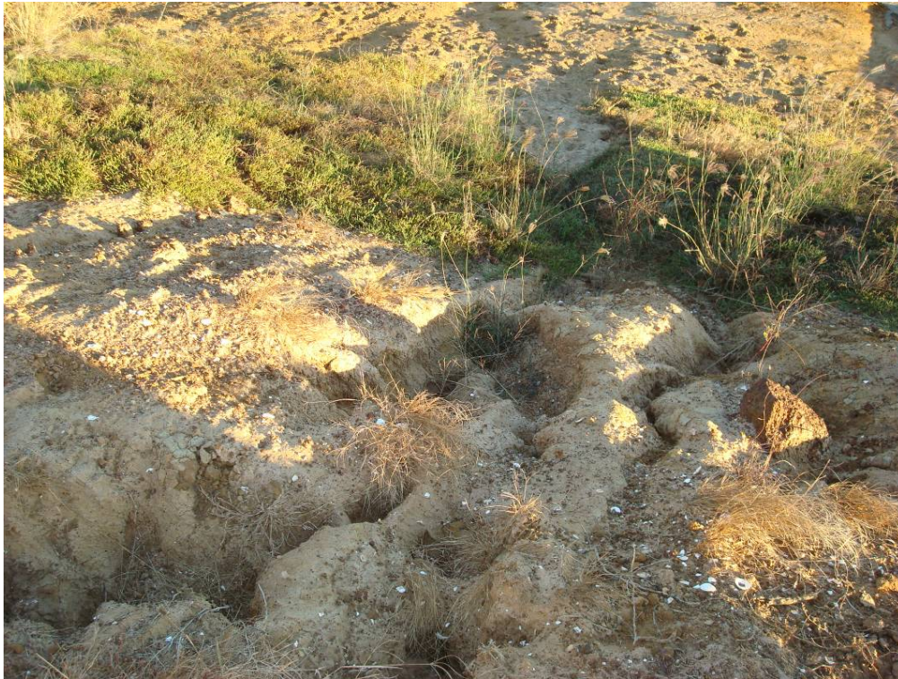
Plate 54 Erosion of dispersive embankment fill at the dredge spoil cells. Photo: Independent Monitor
