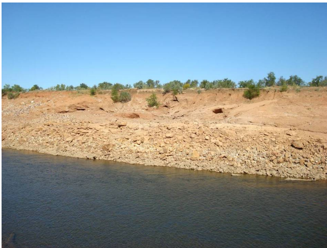
Plate 50 Minor erosion of McArthur diversion batter. Photo: Independent Monitor
