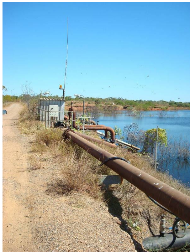
Plate 41 Pumped decant system at WMD. Photo: Independent Monitor.
