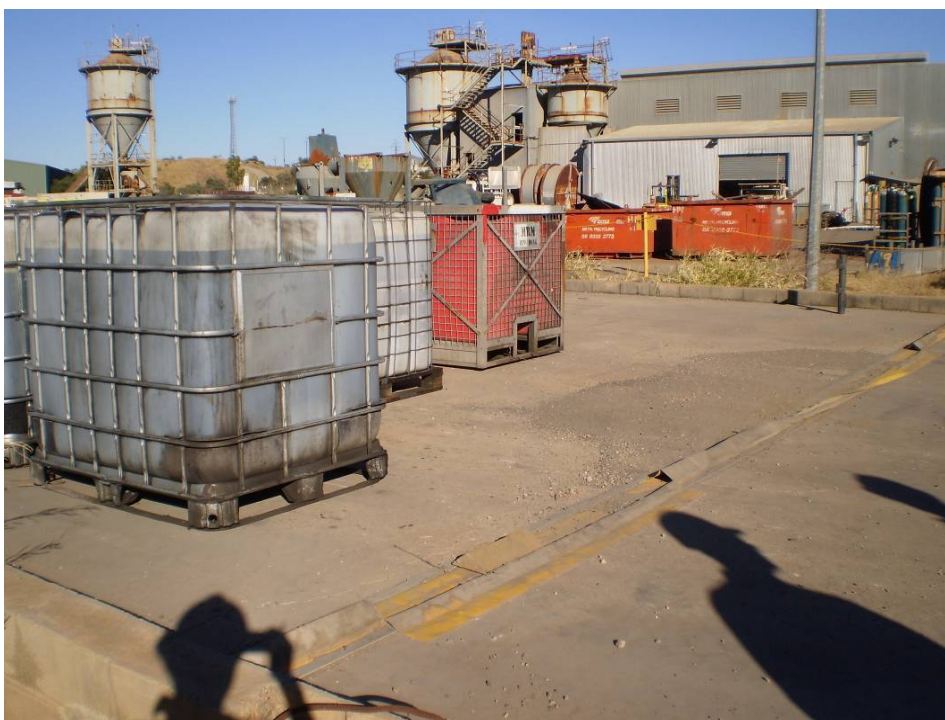
Plate 67 Waste oil stored in IBCs in the store yard. The collapsible bunding shown in the foreground is in need of replacement, and no sump exists in the concrete containment pad. Photo: Independent Monitor
