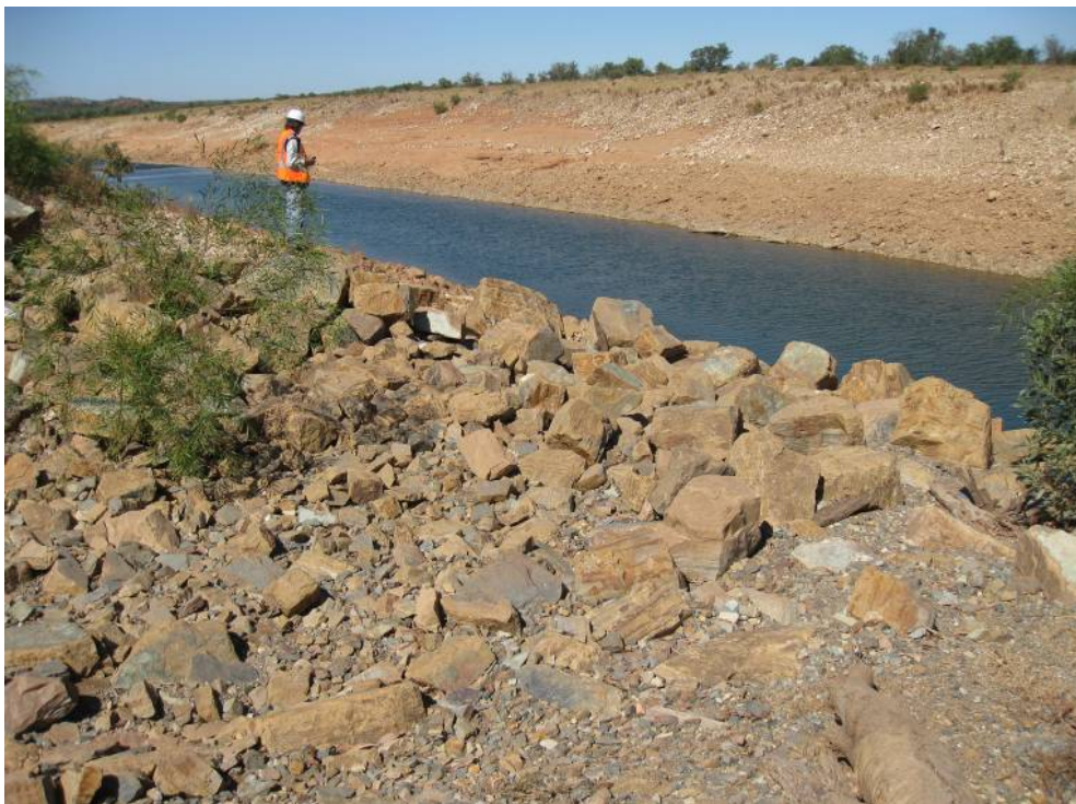
Plate 62 View of rock-lined chute at the diversion channel built as part of 2010 works to address scour along the flow path from the old McArthur River channel to the new diversion channel. Photo: Independent Monitor
