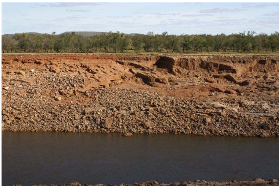
Plate 57 View of eastern batter slope scour at river channel chainage 1750m; taken March 2010. Evidence of significant scour during 2009/2010 wet season flows compared with the 2009 photograph, see Plate 56). Photo: Independent Monitor
