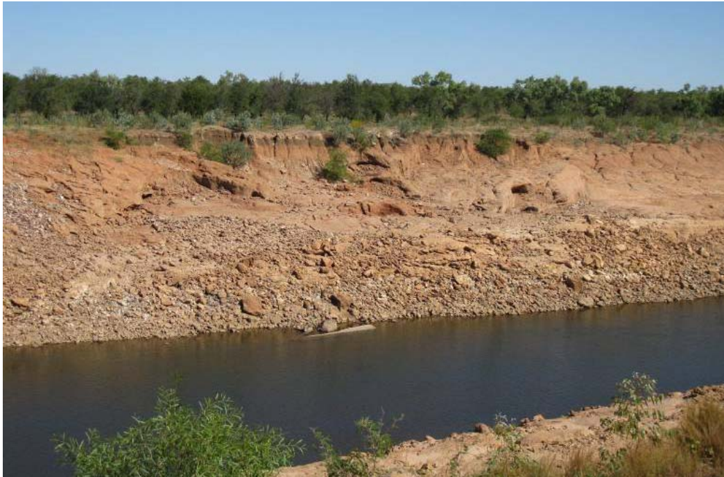
Plate 58 View of eastern batter slope scour at river channel chainage 1750 m; taken June 2011. There is very little change as a result of 2010/2011 wet season flows (compared with 2010 photograph, see Plate 57). Photo: Independent Monitor
