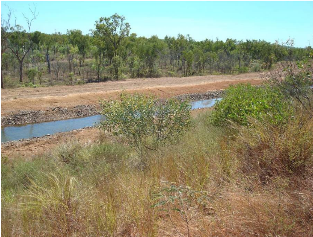
Plate 37 Western seepage collection drain at toe of TSF Cell 2. Photo: Independent Monitor.
