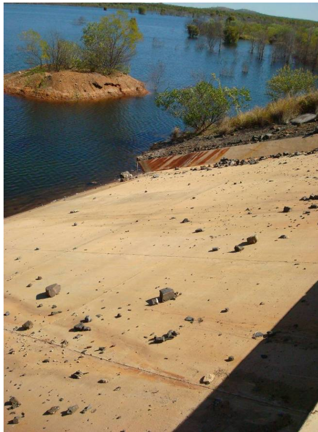
Plate 35 Concrete spillway apron where seepage was noted during previous audit. No seepage was visible during the inspection. Photo: Independent Monitor.
