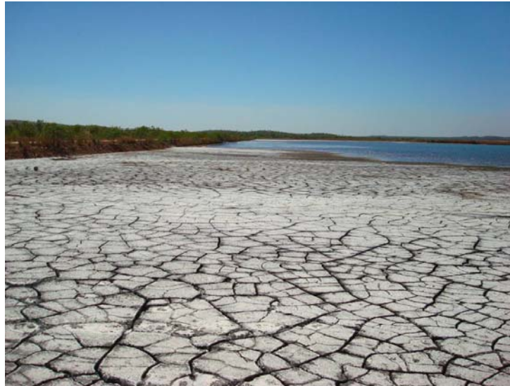
Plate 34 Desiccation of deposited tailings on beaches in TSF Cell 2. Photo: Independent Monitor.
