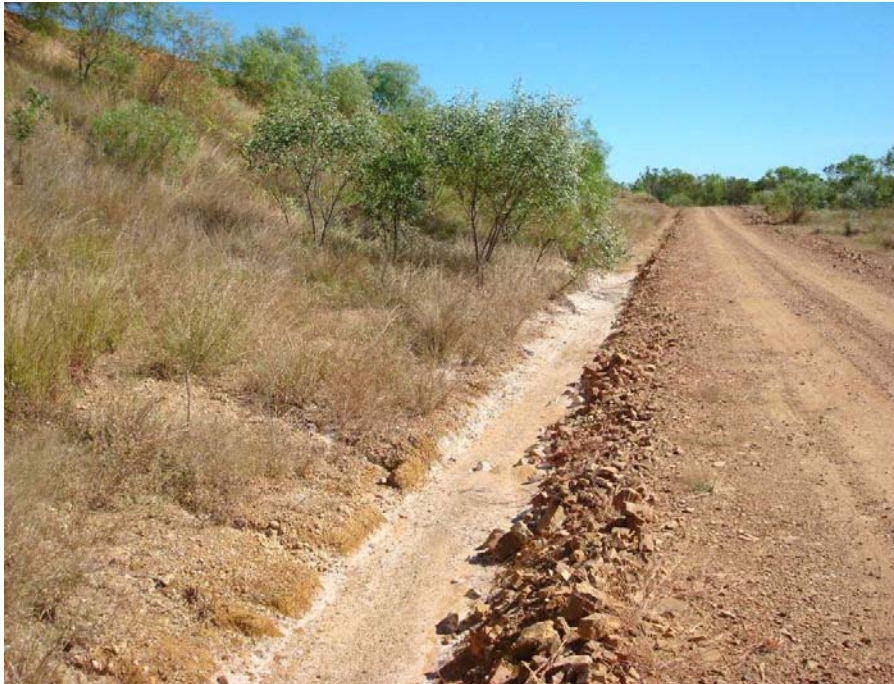
Plate 31 Salt precipitation and seepage on TSF Cell 1 Embankment toe adjacent to Surprise Creek. Photo: Independent Monitor.
