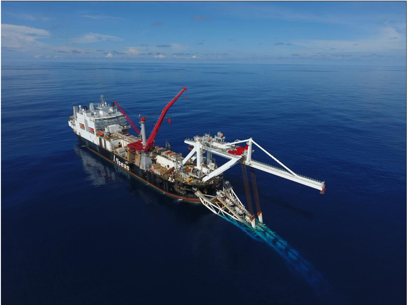
Pipe Laying Vessel 'Audacia'
