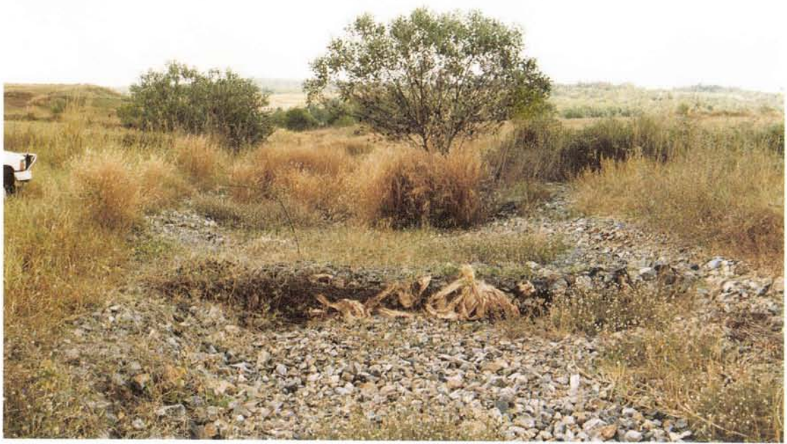
Plate 8.1 White's Heap Drain B looking downstream. Gabion weir constructed 1987.
