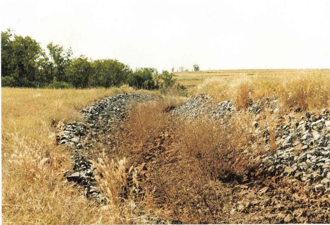
Plate 8.3 Subsidence and backfill in matted drain on Dyson's Open Cut. Created by settlement of fill. May 1988.
