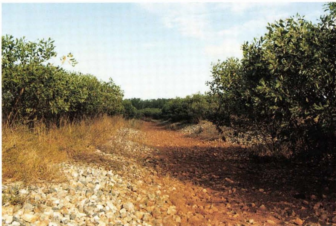
Plate 8.8 Close up view of main drain on the Tailings Dam area, showing developing tree belts and infilling of rip- rap voids with fine material. May 1988.
