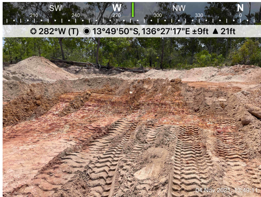
Test Hole in Laterised soils
